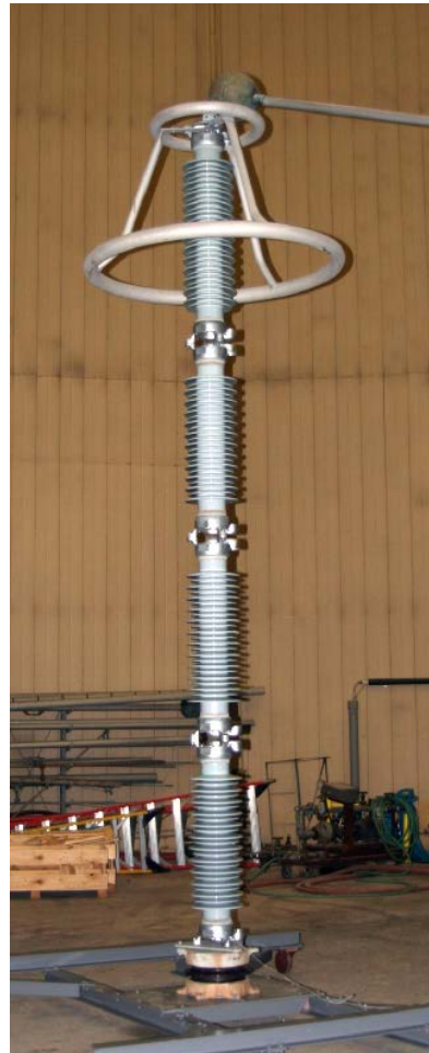
Figure 1. Arrester installed for RIV test
