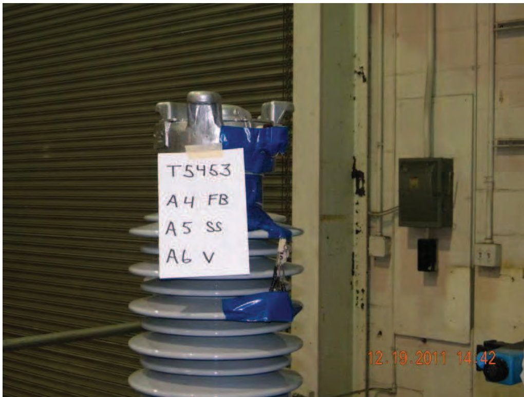
Figure 3. Accelerometer Locations A4, A5 and A6
