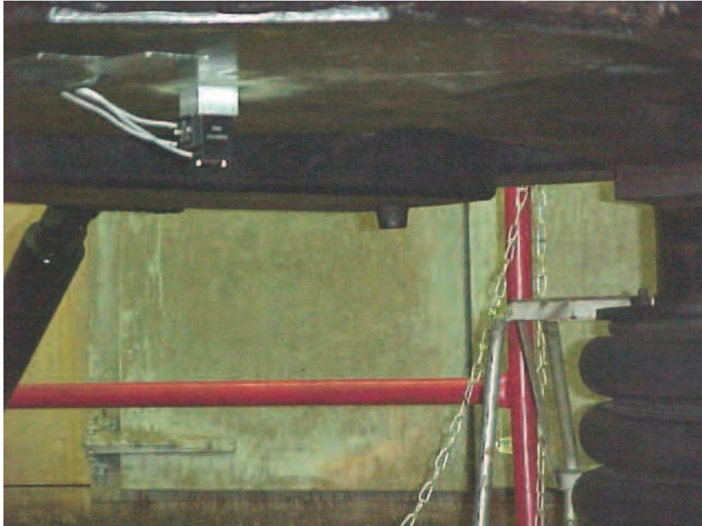
Figure 2. Accelerometer Locations A1, A2 and A3
